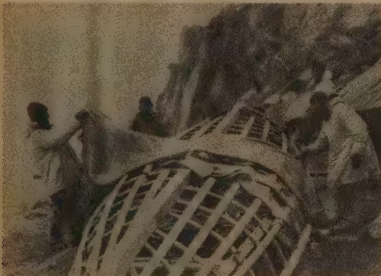
Arctic boatbuilders apply the ideal covering — split walrus hide.
